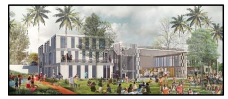
containers as "building blocks" to create an energy- and cost-efficient structure. These components will be blended with more traditional modular construction to create a large multi-purpose pavilion and various common areas in the building.
