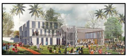
containers as "building blocks" to create an energy- and cost-efficient structure. These components will be blended with more traditional modular construction to create a large multi-purpose pavilion and various common areas in the building.
